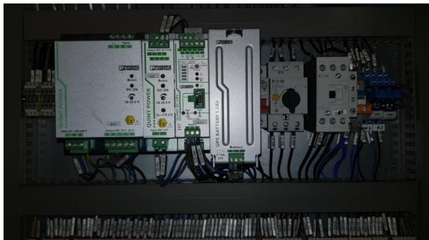
**Fig. 9 The power supply of the LCP**
